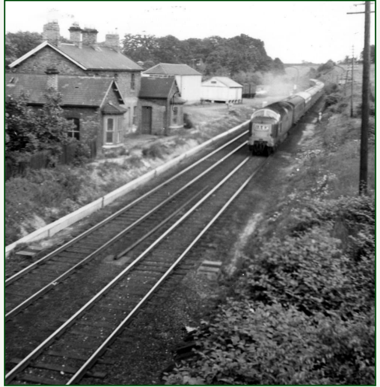
Plawsworth Station, platform removed, early 1960s Photo courtesy of Roy Lambeth
