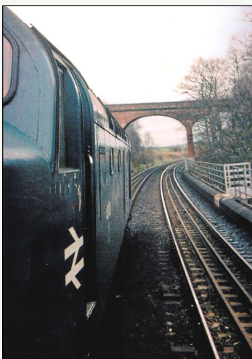
Train heading southbound from old Plawsworth Station site, under a viaduct (now demolished), 1983 © Robert Patterson (Flickr)
