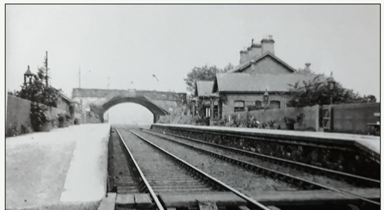
Plawsworth Station and Wheatleywell Lane road bridge Source and date unknown
